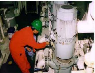
Wireless monitoring the temp and vibration without circuiter
